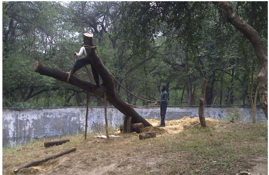
Placing the tree inside the pit
